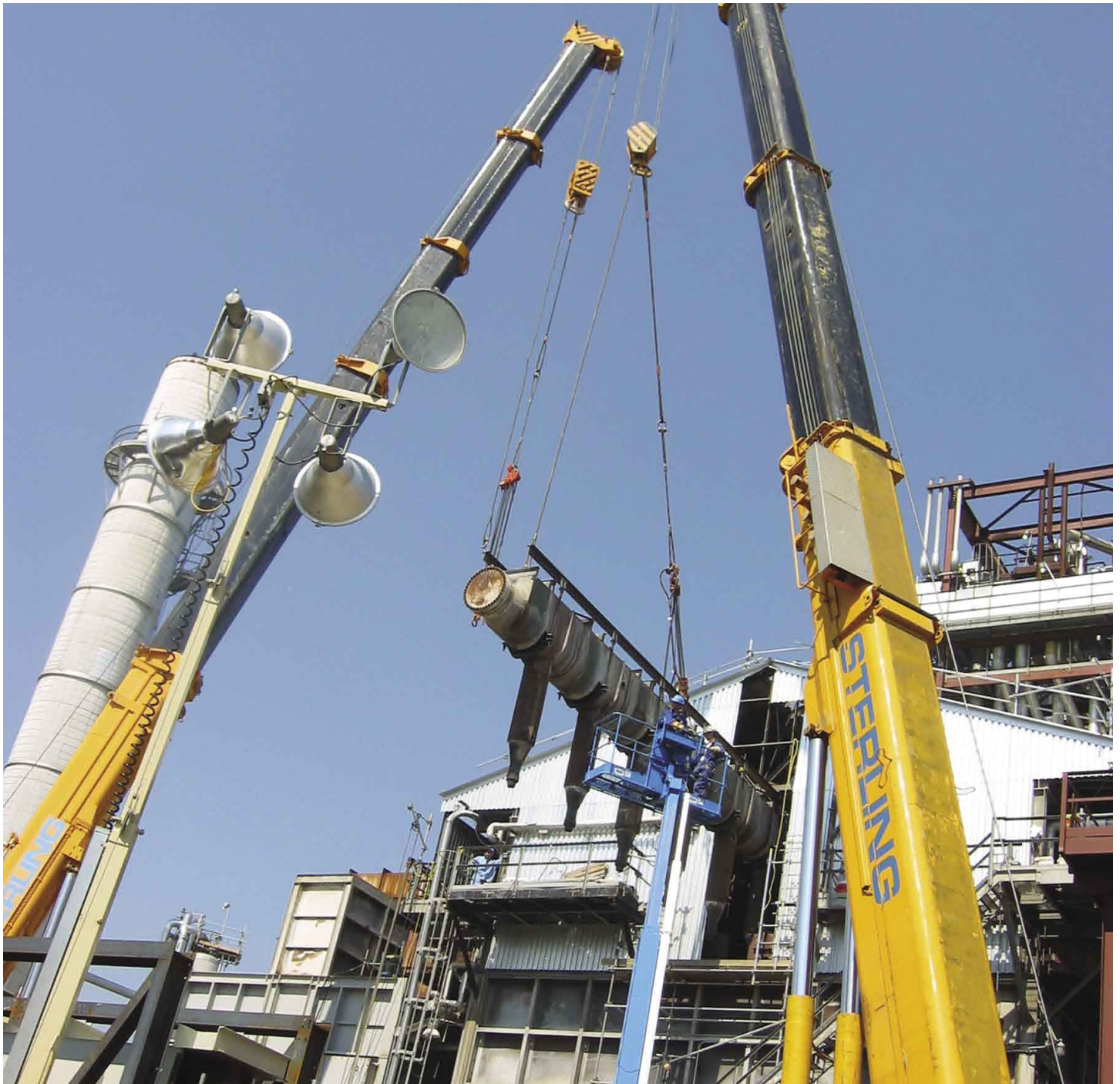
Engineering of rail system and removal of reformer overhead transfer line performed by Edmonton Exchanger at client site.
